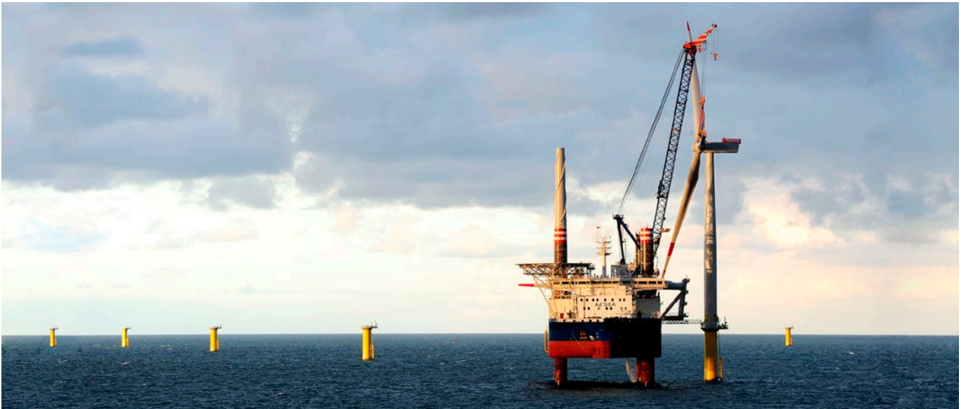
Installation of first wind turbines at Borkum Riffgrund 1. ©DONG Energy
